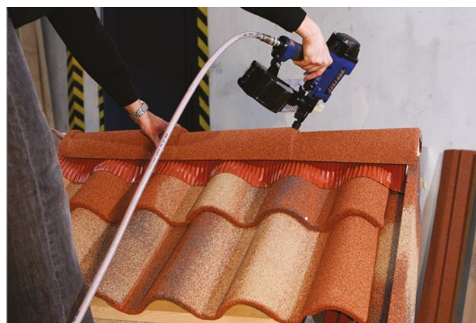
Fixing of ridges
